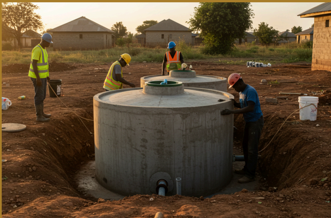
Workers installing large underground water storage tanks in a rural setting.
