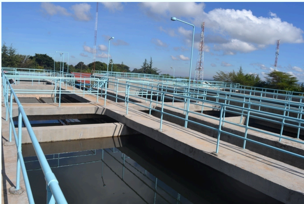
The image showcases Nawasco's two water supply infrastructures near Fairmount Mount Kenya Safari Club. The older treatment facility produces 1,000m 3 /day, while the newer facility has a capacity of 11,000m 3 /day.
